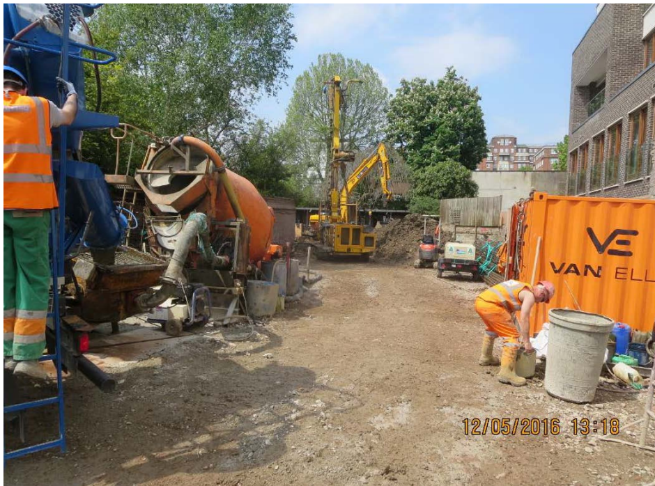
Previous building on site prior to demolition (top) and site as of May 2016 with previous building on site completely demolished (bottom).
