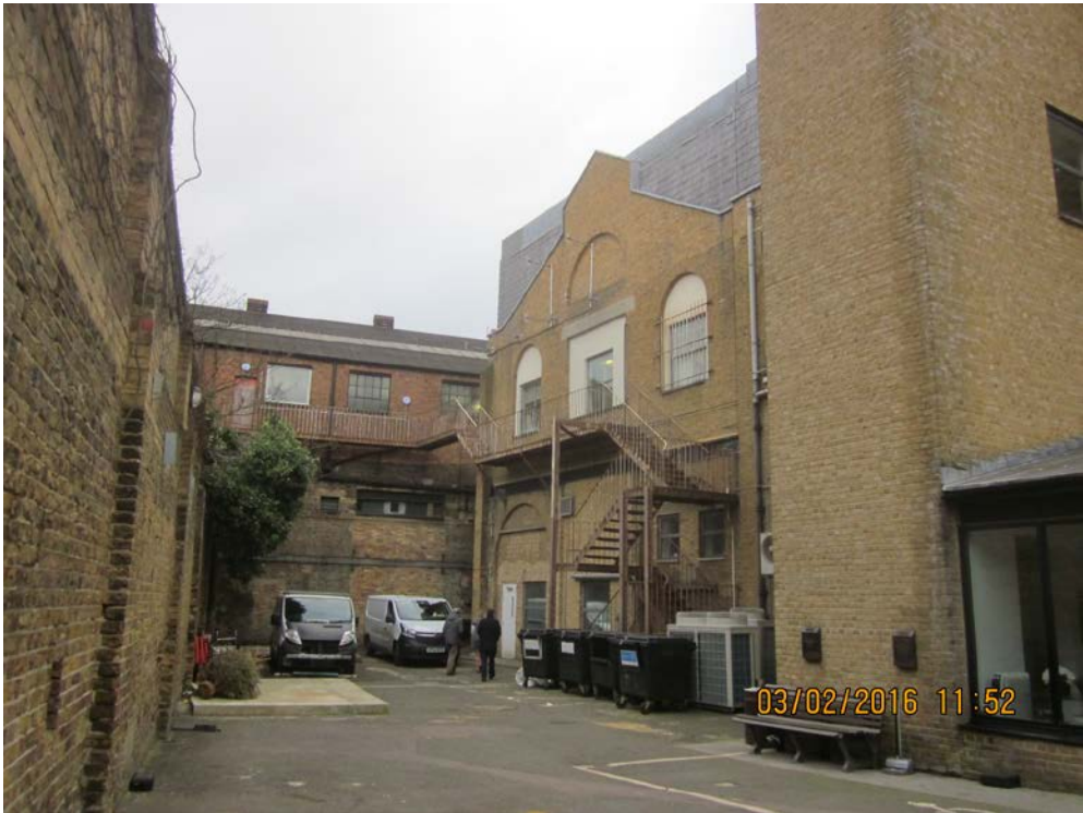
Rear of 25 Eccleston Place
