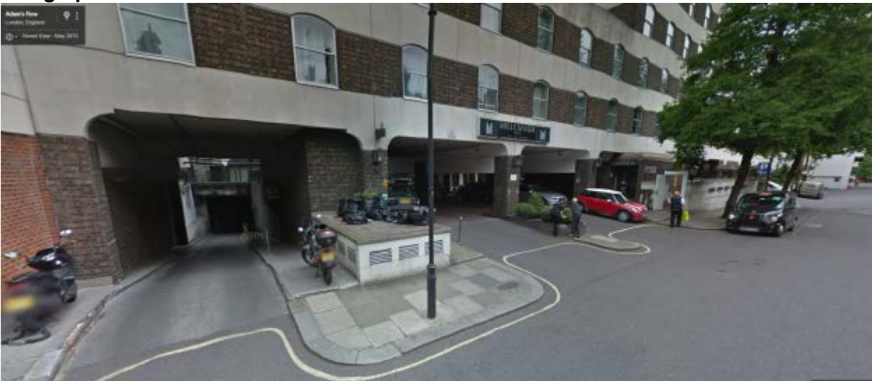
Photograph 4. View of Adam's Row from the West.
